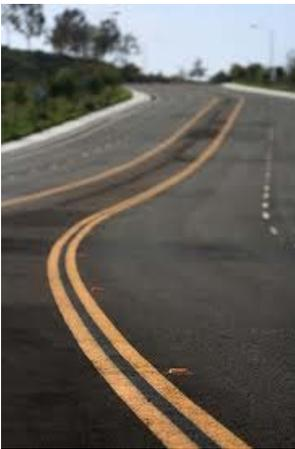
Signing and striping are used to help reduce speeds in residential areas. Striping creates narrow lanes that give the illusion of a narrow street. Signing enforces speed reduction with the use of speed limit signs and/or neighborhood signs.
