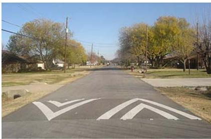
Speed humps are rounded raised areas placed across the road. They are generally 12 feet long (in the direction of travel), 3 to 3 ½ inches high, parabolic in shape, and have a crossing speed of 15-20 mph. speed humps on roadways with multiple lanes should have a sinusoidal profile. When placed on a street with rolled curbs or no curbs, bollards are placed at the ends of the
